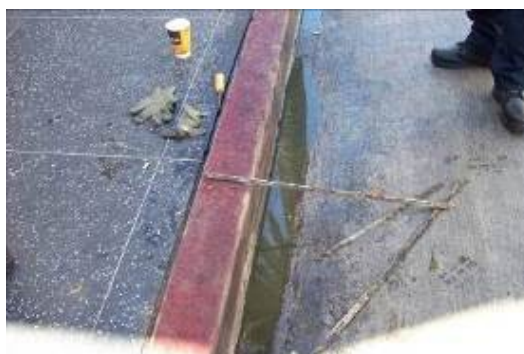
Kyle's Illegal Renovation of the Sidewalk
